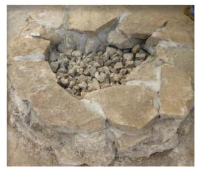
Once the base was built we laid bottles inside the opening and stuffed a mixture of clay, sawdust and water in between the bottles. We then covered this layer with sand and leveled it. This acts as an insulation layer to keep the base from soaking up the heat of the oven.
