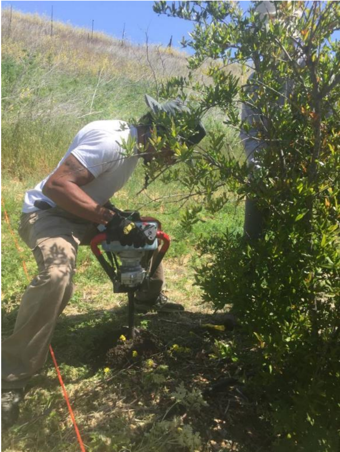
Drilling first before inserting the stakes.
